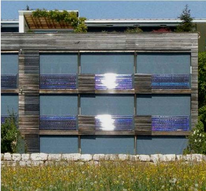
Façade integrated evacuated solar collectors (Sunny Woods, arch. Beat Kämpfen)
